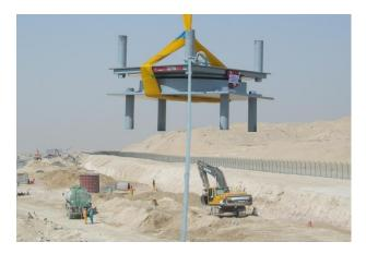
Robust transportation devices are fitted to all bearings to ensure that the movable components are maintained in their correct relative positions before and during installation. These temporary fixing devices are normally finished in red paint and shall be removed after installation.
