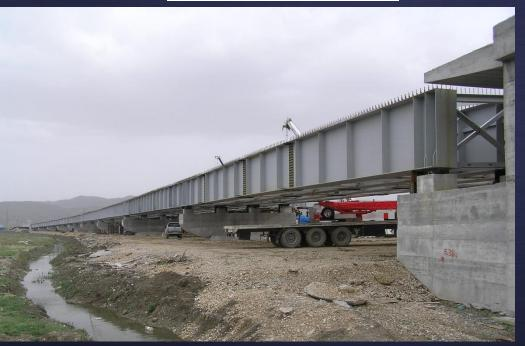
n.112 spherical bearings according to EN1337 n.8 elastic restraints + shock transmitters
